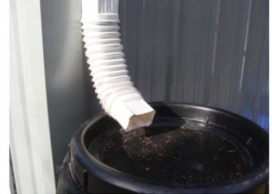
Slip the downspout adapter onto your downspout and direct the other end onto the top of the barrel
